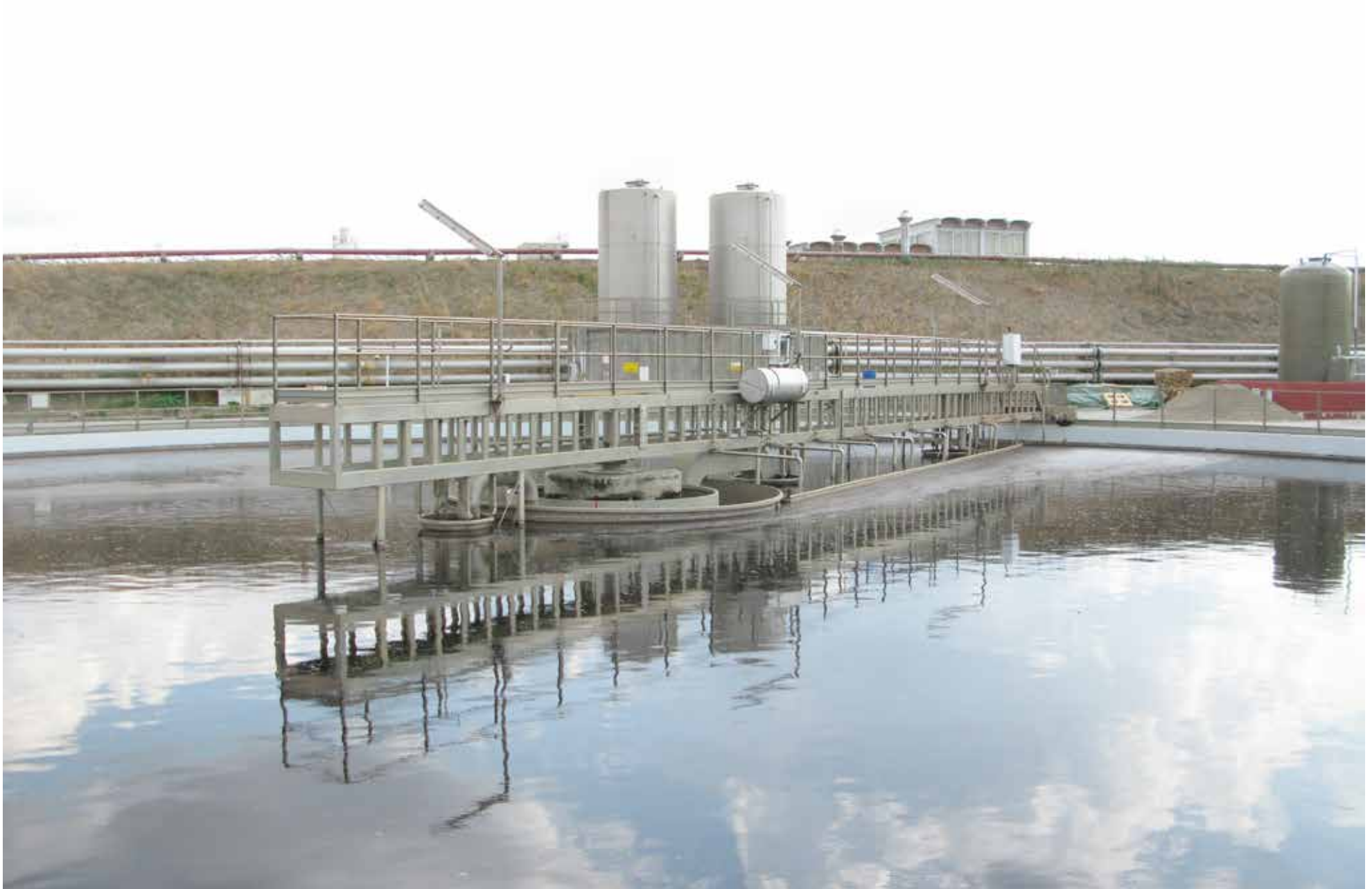
Stille work in progress il depuratore / the water treatment plant
