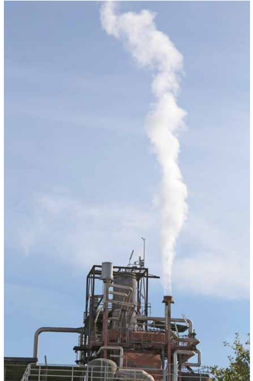
Stille work in progress Ecoespanso
