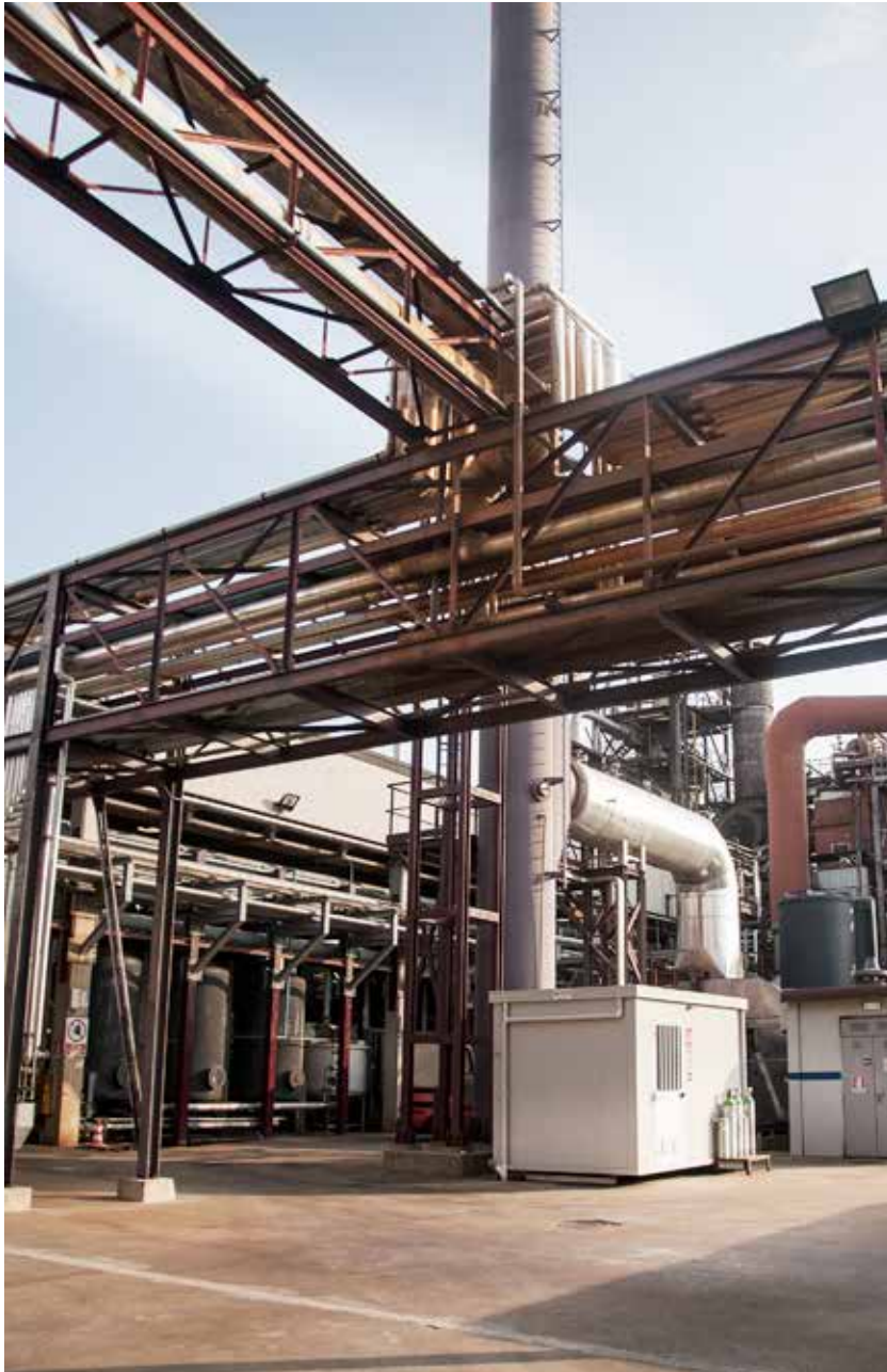
Stille work in progress Ecoespanso
