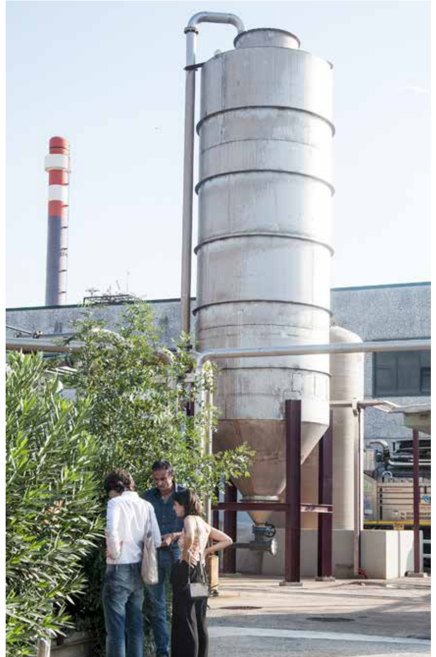
Stille work in progress Ecoespanso
